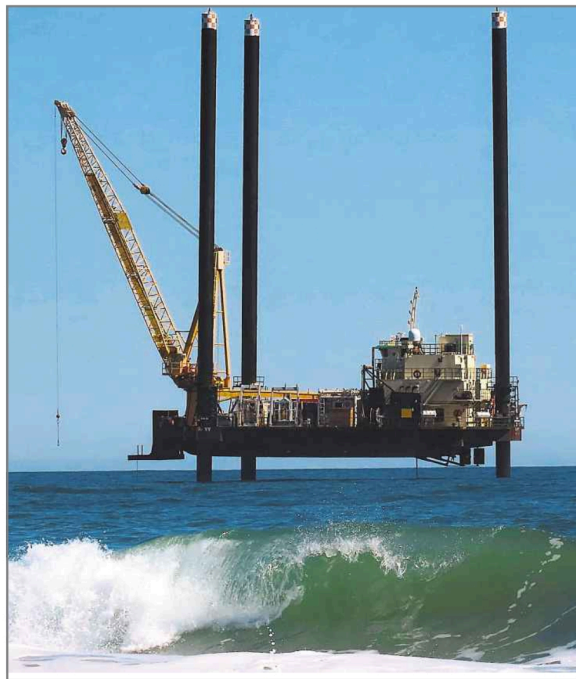
A barge in the Atlantic is seen in March off Smith Point County Park in Shirley during work on Orsted's other project, Sunrise Wind.
